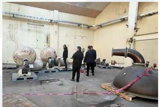
Image from Cadbury demolition - See Mana Ahurea update (page 3)
